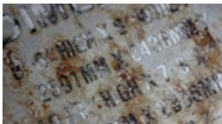
Road Salt Corrosion Damage
